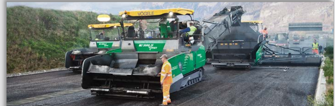
Feeding pavers when working "hot to hot"
