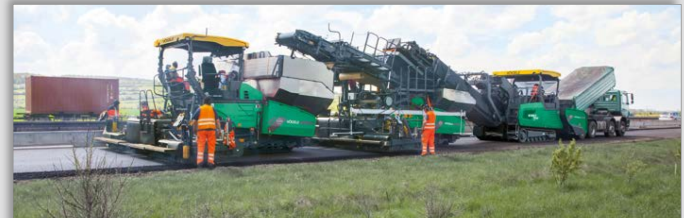
Feeding pavers in an InLine Pave train
