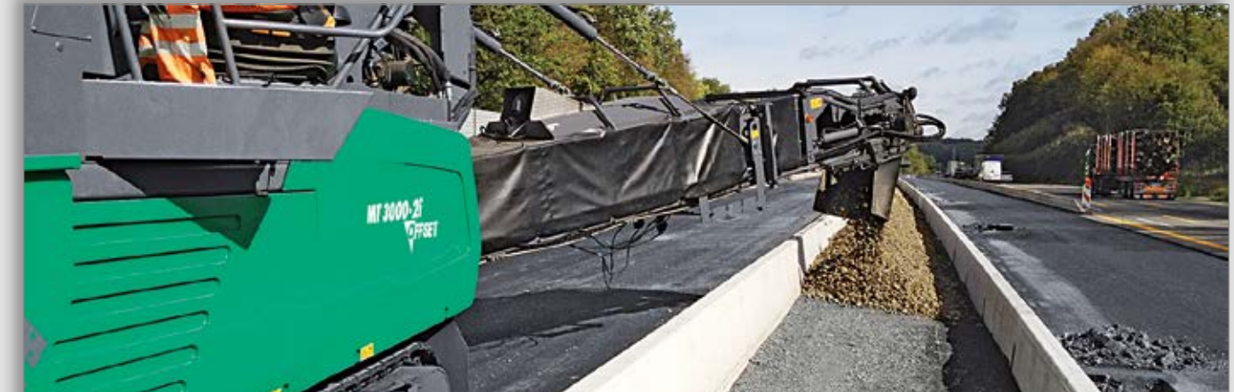
Filling cavities between safety barriers
