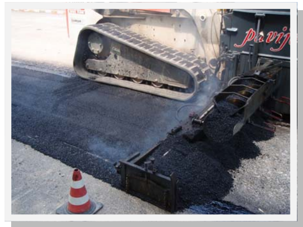
MG7 paving a shoulder.
