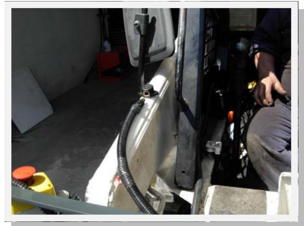
Power connection to skidloader (MG6 & MG7).
