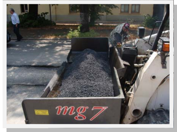
MG7 paving a shoulder.
