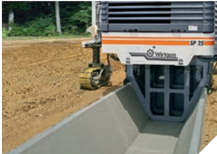
◀ Paving a large water canal
