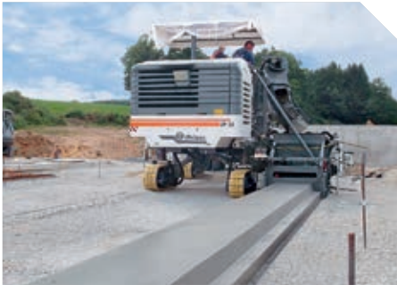
▼ Pouring a large special profile
