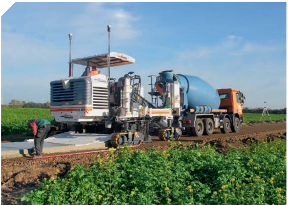
◀ Paving a large water canal
