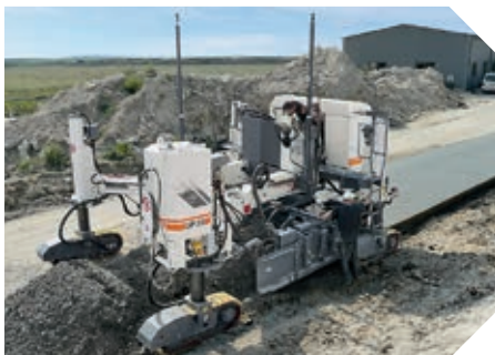
▲ Paving a 8' 2" (2.5 m) wide main road using 3D control Precise paving of a 9' 10" (3.0 m) wide agricultural road using the Wirtgen AutoPilot ▶
