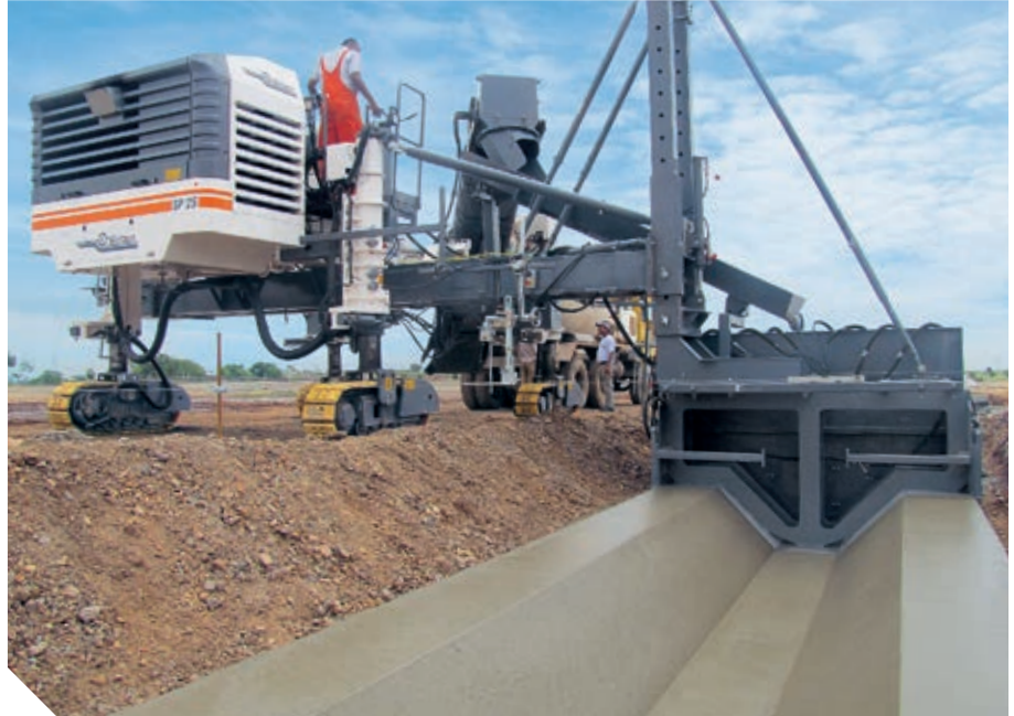
▲ Paving a rainwater gutter along a steep slope from the right ...
