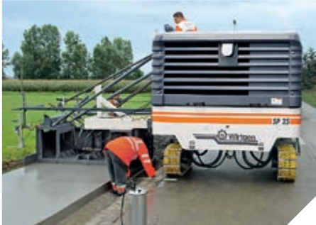
▲ Paving a 8' 2" (2.5 m) wide bicycle path
