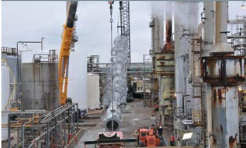
In just eight months, Turner Industries Group completed the design, fabrication, delivery and installation of a 100-ton, 206-foot-long distillation column, including a long, incident-free haul from Decatur, Ala., to Houston.
