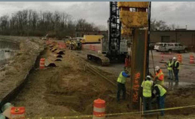
On its first prime contract with the USACE, Kwest Group safely dealt with overhead utilities and underground conflicts while constructing 2,600 traversing feet of customized reinforced concrete floodwalls partially located within 25 feet of surrounding businesses.
