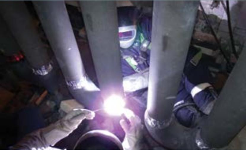
Starcon International completed the highly specialized welding necessary to re-tube furnaces for a chemical company, achieving 3,000 welds annually at a 98 percent acceptance rate.
