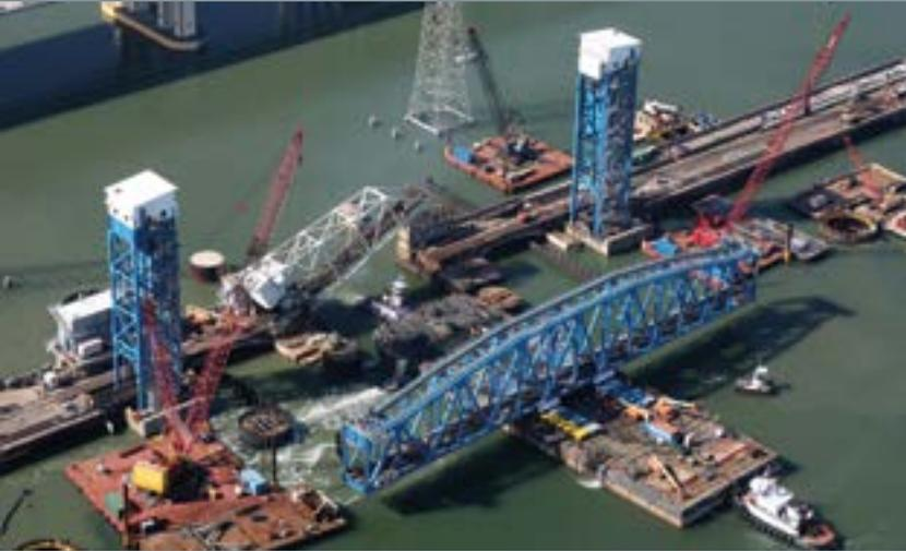
Cianbro and Brasfield & Gorrie worked around the clock to fabricate and erect this 382-foot-long, single-track vertical lift railroad bridge in 32 months without disrupting bridge and waterway operations.
