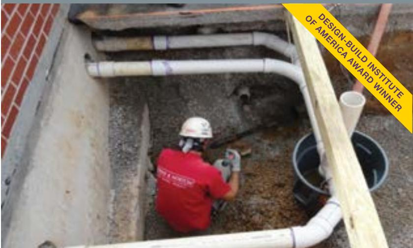
Early Services leveraged its design-build expertise to replace 155 feet of deteriorating sewer pipe in just two days using an innovative pipe bursting technique to save the owner more than \$100,000.
