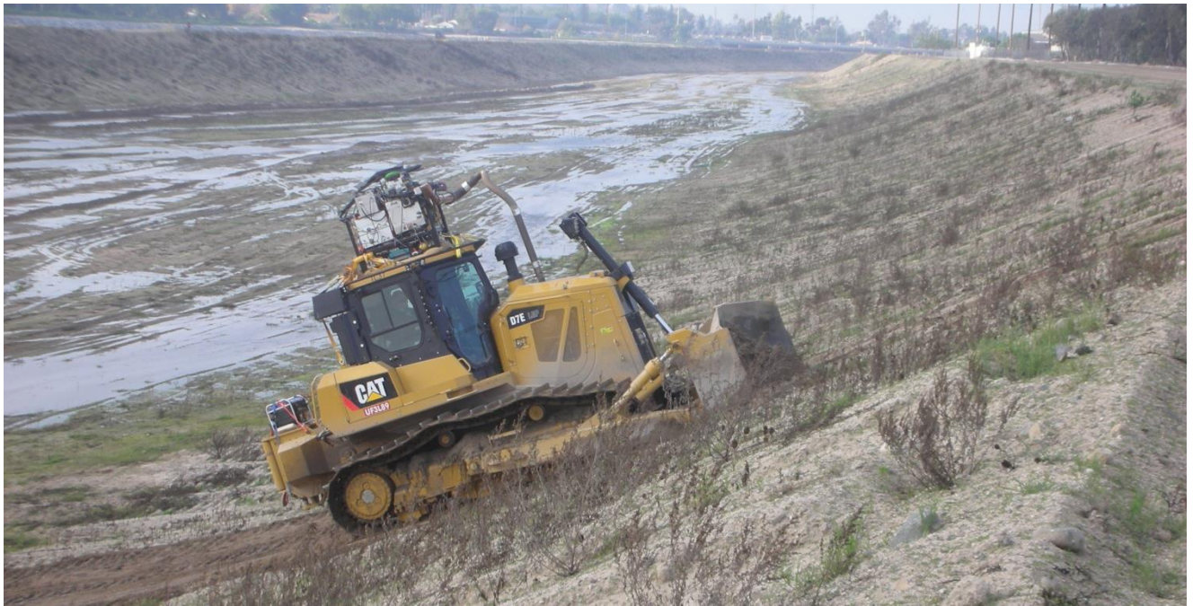
Figure 5-23 OC's D7E performing slope cleaning in-service push river maintenance.
