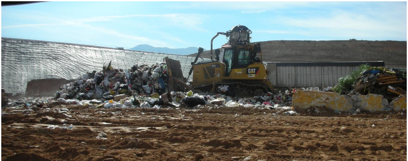
Figure 5-21 WM's D7E in-service trash push at El Sobrante landfill near Corona, CA.
