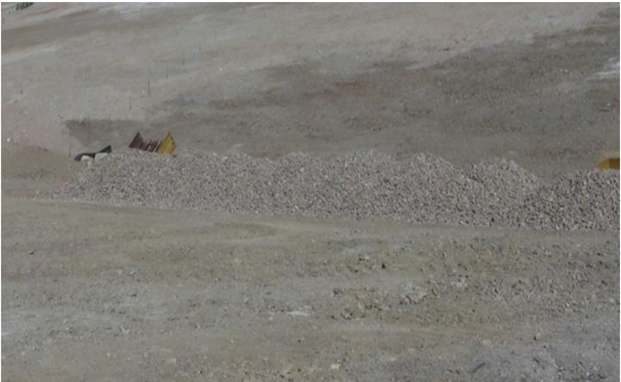
Figure 5-2 Delivery of eight loads of three inch minus rock (104 tons)
