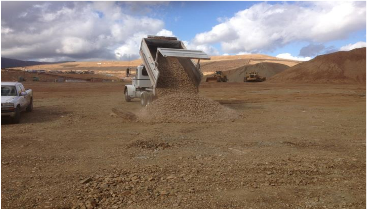
Figure 5-1 Delivery of one load of three inch minus rock (~13 tons)
