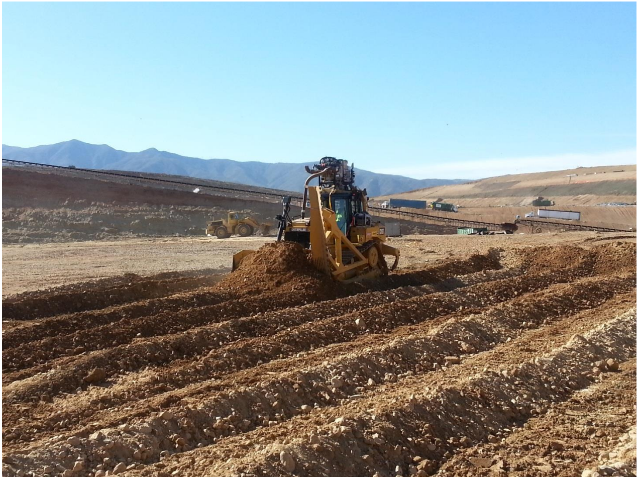
Figure 5-20 In-service dirt and 6in minus rock pile pushing – D6T.
