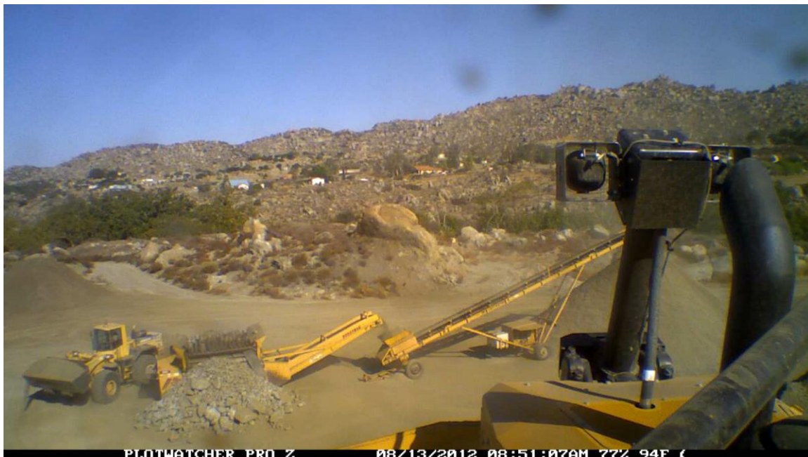
Figure A6 RC’s daily operation, the D7E is now on the top of the mixture pile.
