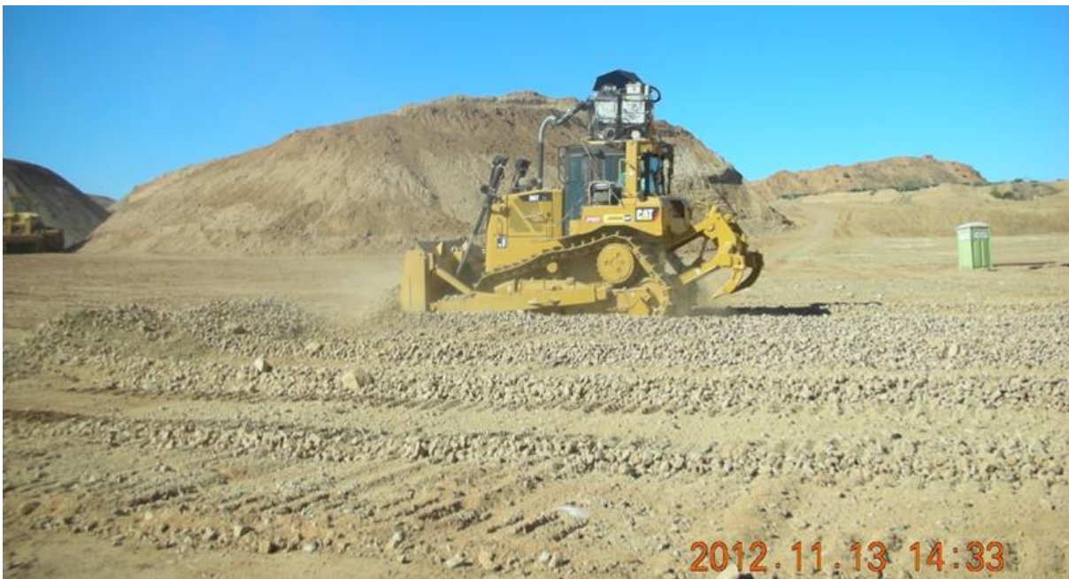
Figure 5-5 D6T 30 meter push after the 4th pass of the bulldozer
