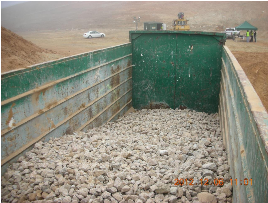
Figure 5-14 Pull test approach showing 3 loads of 3" minus rock in container (#3 bin D8T)
