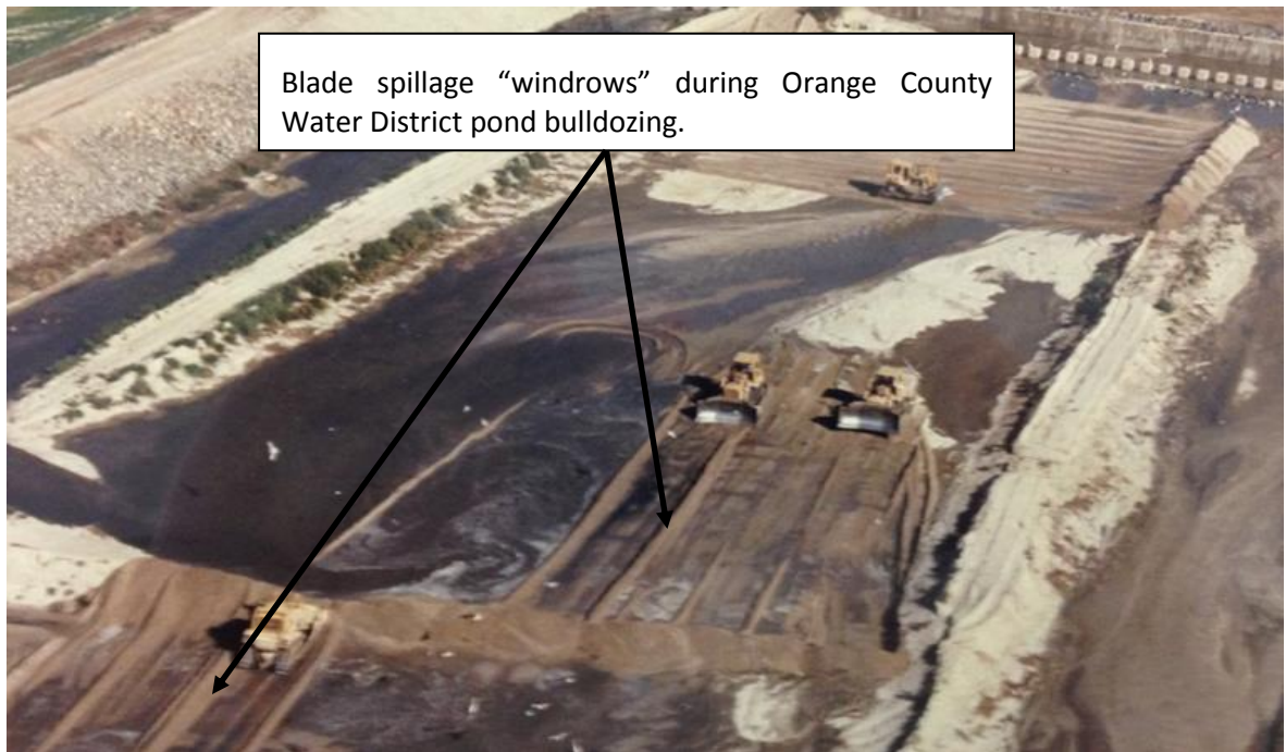
Figure 5-8 Blade spillage or "windrows" during OC bulldozing
