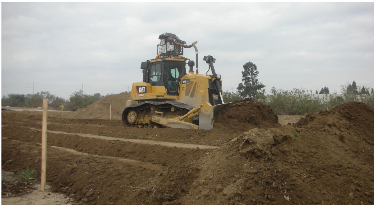
Figure 5-24 OC's D7E performing 50'x50' pad cut in-service test.
