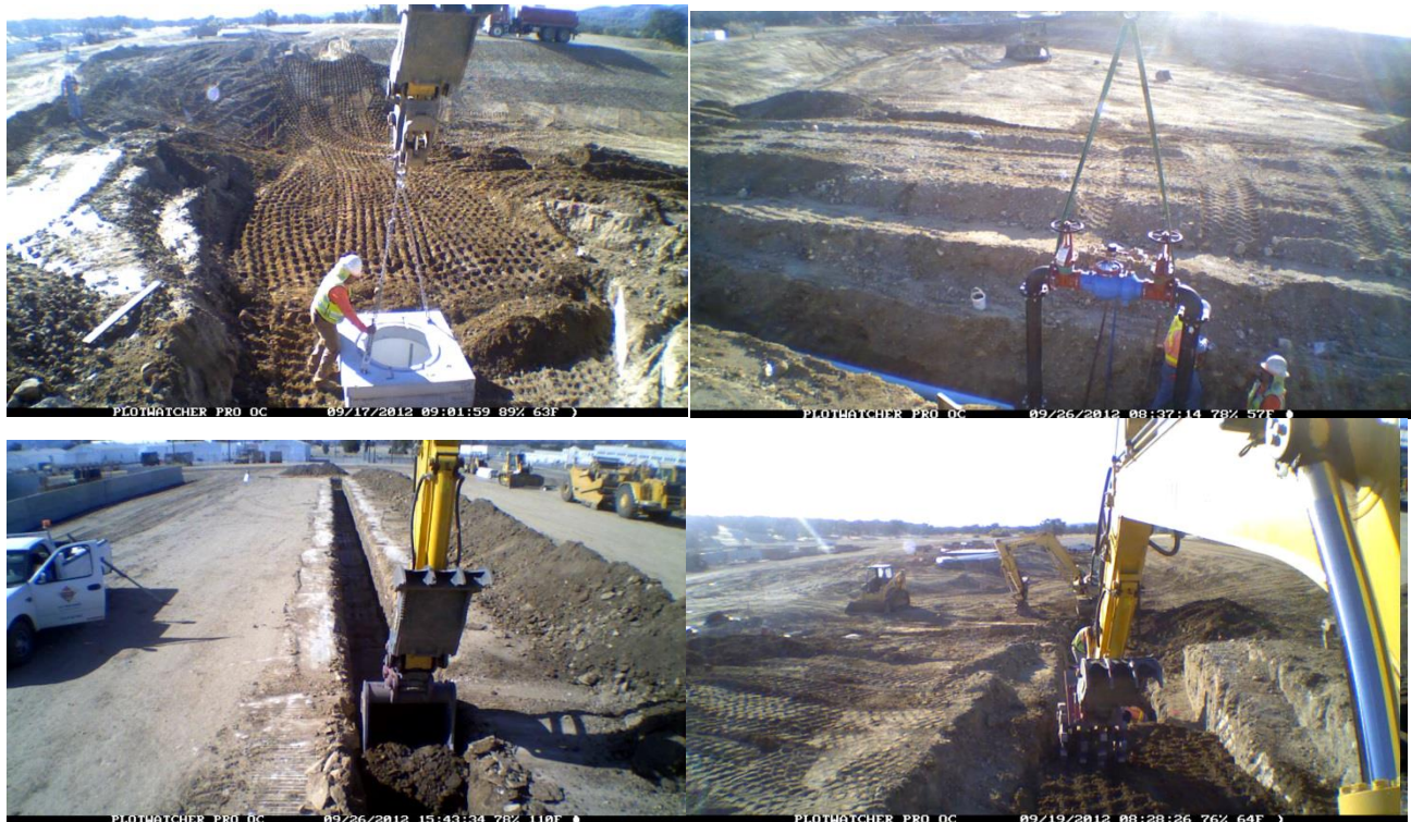
Figure 4-24 Activity time lapse video from the excavator for various operations
