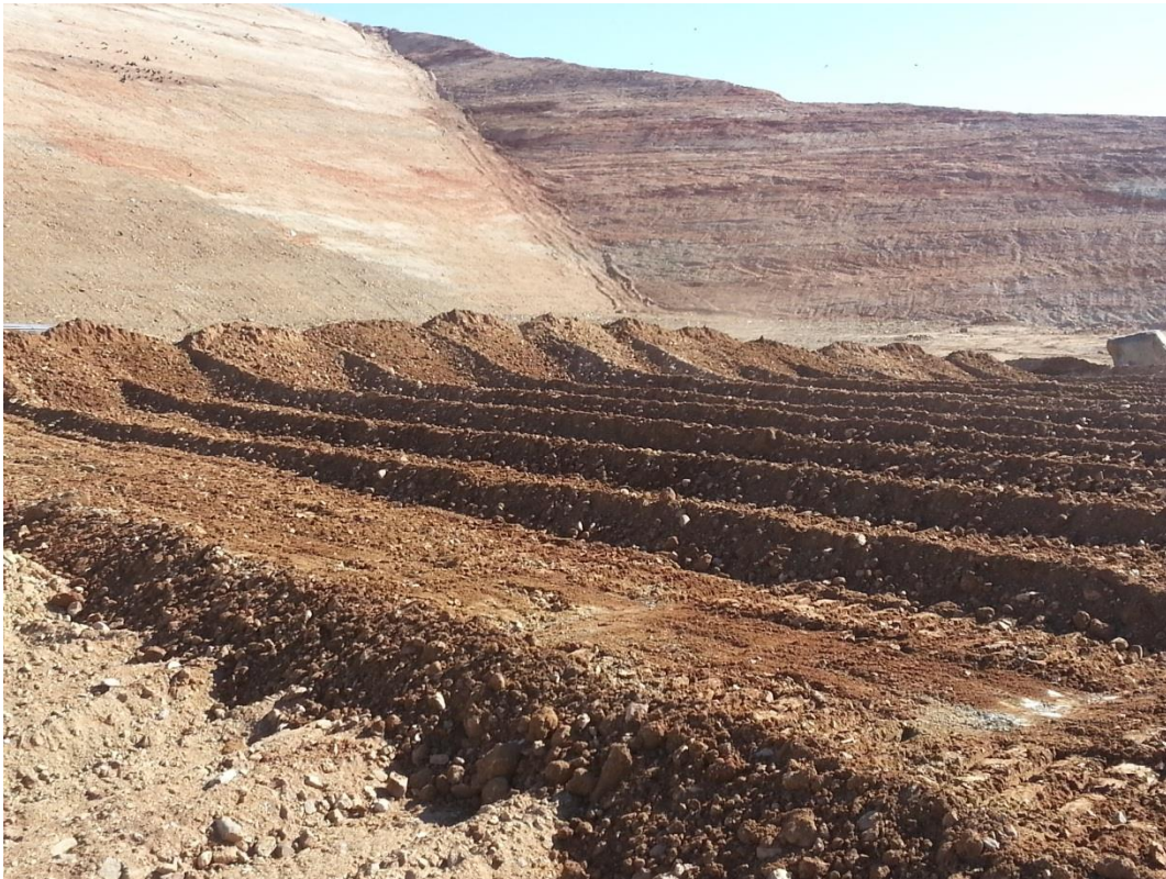
Figure 5-7 Massive windrows (~3 ft high) after a few full blade pushes.
