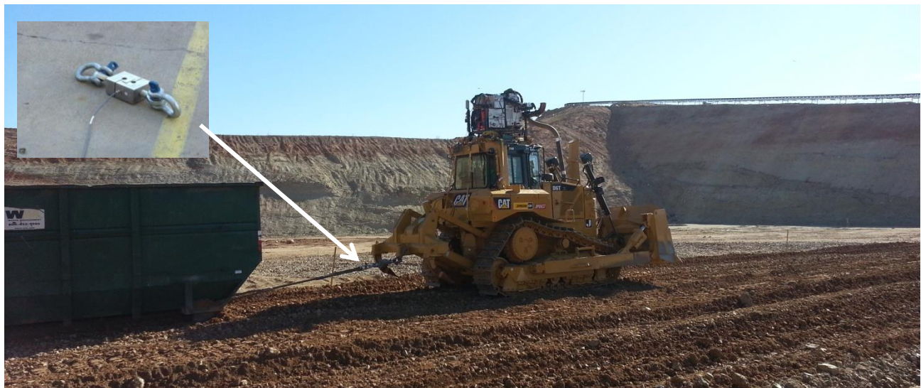
Figure 5-13 Pull test approach with D6T and container loaded with 13 tons of rock
