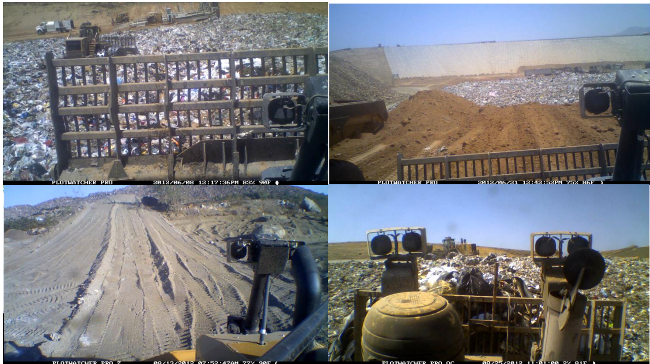
Figure 4-9 Activity time lapse video from the bulldozer for various operations
