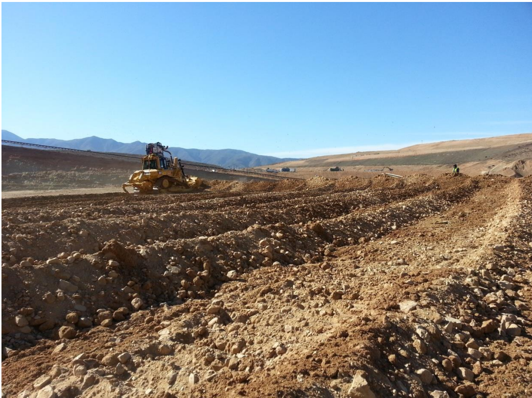
Figure 5-6 D6T Rock Pile pushes showing windrow formation.
