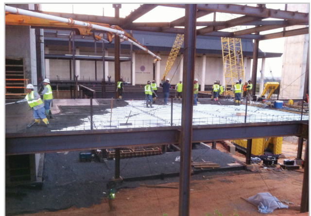
working with DeckMaster - "just mix and pump"
