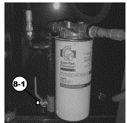
8 - fuel supply valve and filter
